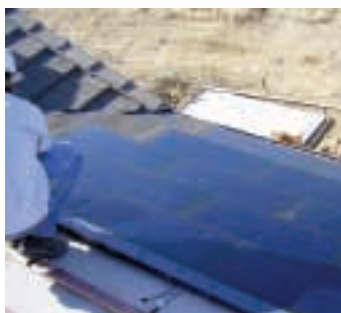
Open Energy solar panels being installed
